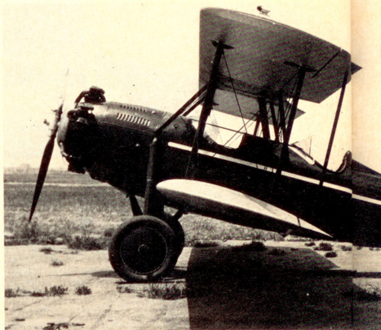
The most popular model in the Spartan biplane line was the C3-165 with the 165-hp Wright J-6-5 Whirlwind engine. Note the completely redesigned landing gear.
